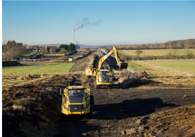
Removal of MCJ line, Grendon Underwood
