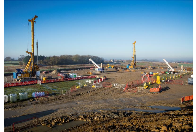
Piling to Perry Hill Overbridge, Twyford
