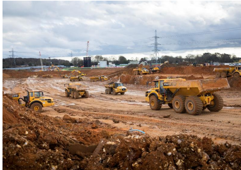
Excavation to South Heath Cutting, Gt Missenden
