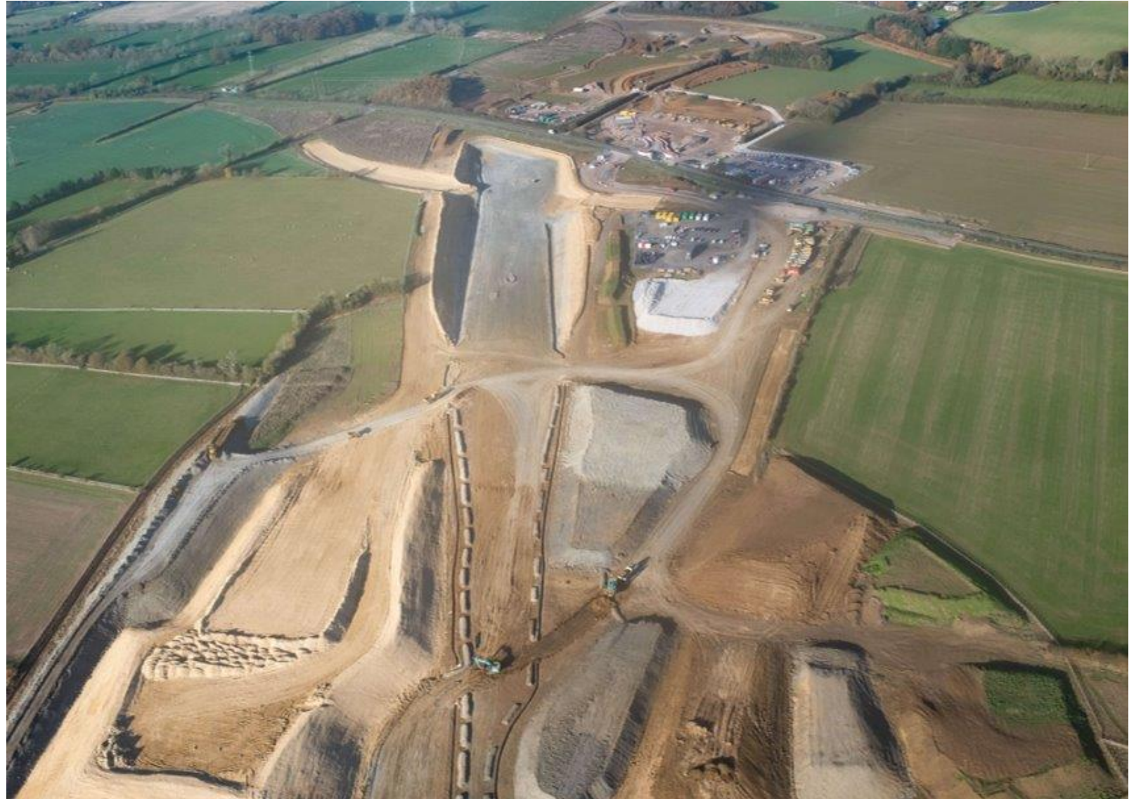
Initial Excavation to Turweston Cutting
